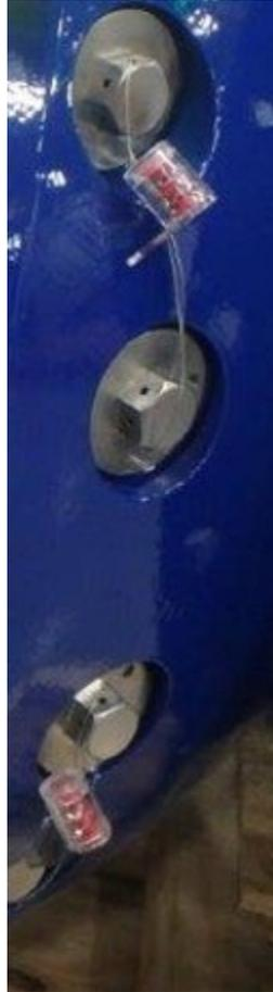
**Figure 8.5—Seal wire on meter body**
