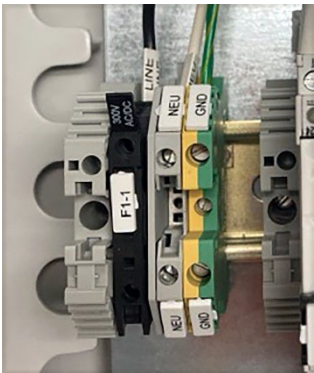
Figure 4.6—AC power connection in HCC2 enclosure
