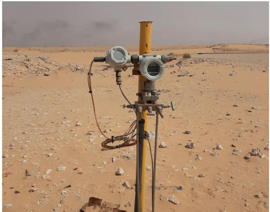
**NUFLO Scanner flow computers have enabled reliable remote monitoring of gas lift injection in a harsh environment.**
